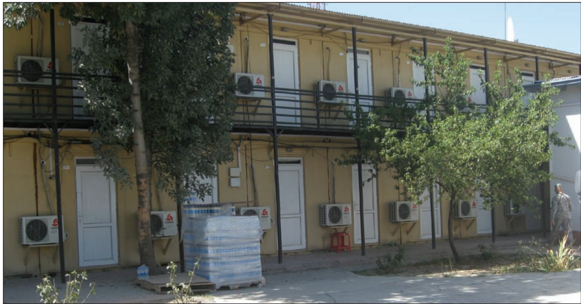
"Hotel California," above left, at Camp Eggers was built by welding 36 shipping containers together.
