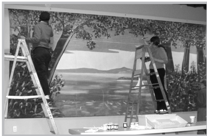
Restoration work takes place on the Painted Theater Curtain recently installed as a back drop in the Danville Town Hall.
