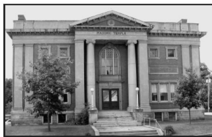
Masonic Temple 115 Eastern Ave., St. Johnsbury, VT
