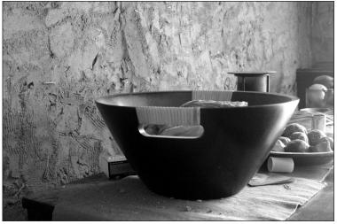
The insulation in O'Hagin's home is partially by means of hay bales covered with adobe. They separate the inside temperature from the outside, and they serve as a heat sink or thermal mass as the shines on them during the hours of daylight. They provide a wonderful organic background, perhaps reminiscent of her early life in the American southwest.
