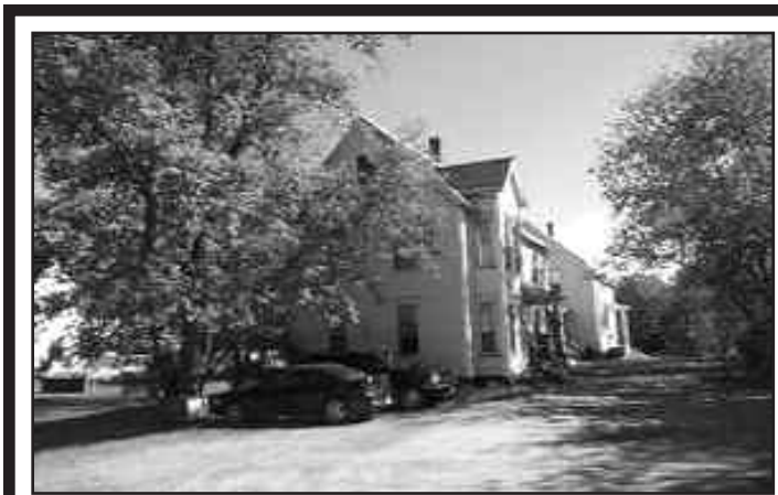
St. Johnsbury: Well kept five-unit building (possible sixth unit) with good numbers on Elm Street. Full basement. Lots of parking. $199,900
