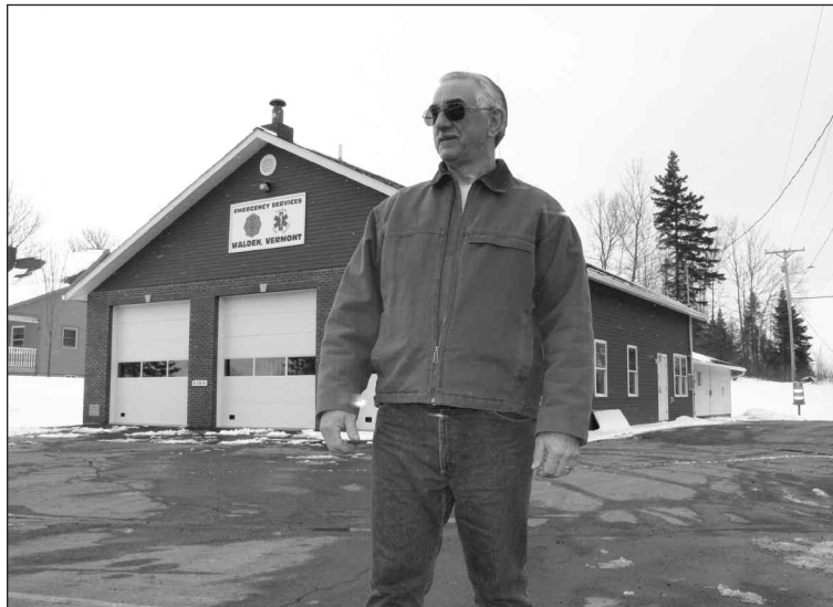
Dennis Larrabee was overseer of the 2005 construction of the Emergency Services Building at Walden Heights. The project was completed on time and on budget with labor from the Caledonia County Work Camp. Larrabee understands the value of the work to the town and the value of the experience to the inmates. He continues to praise their work and remains in contact with one of the inmates who worked on the project last summer.
