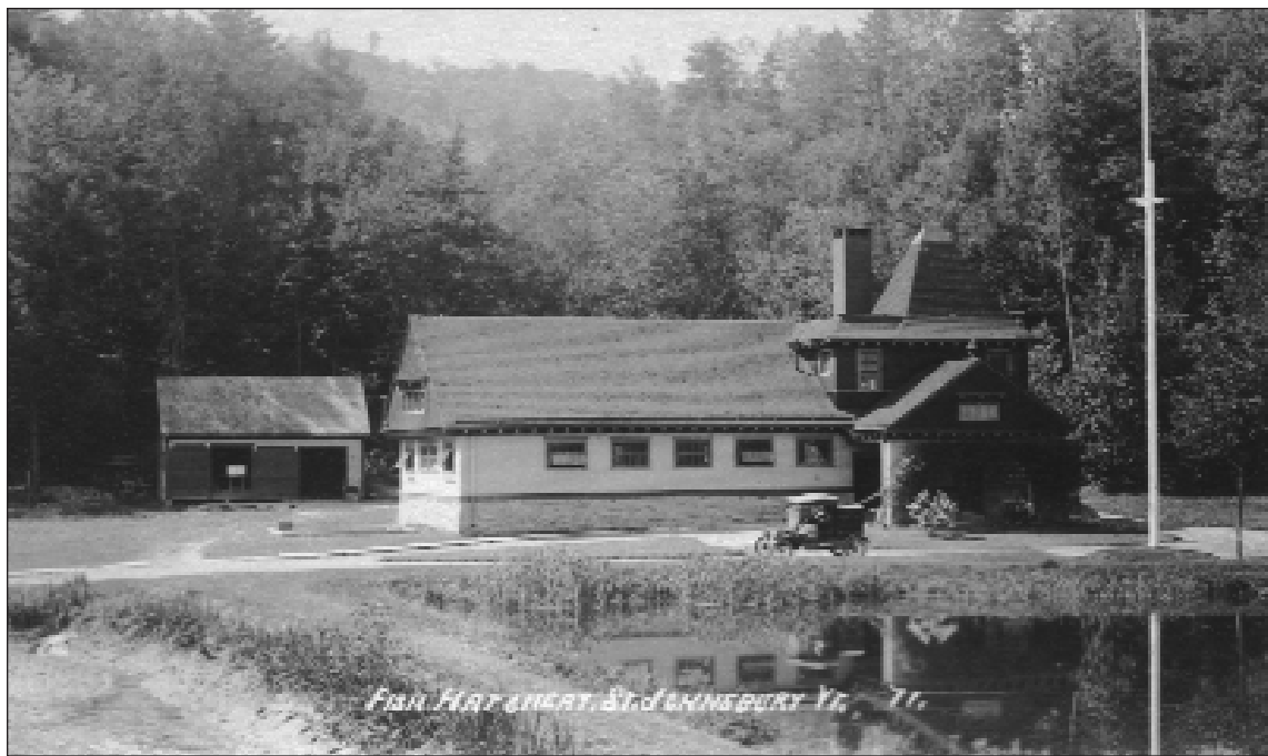
A dwelling for the superintendent, a barn, the hatchery building and an icehouse for fish food (all painted white with green trim) were constructed in 1894.
